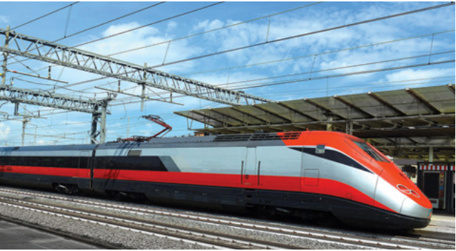
Voltage support systems in railways traction lines
