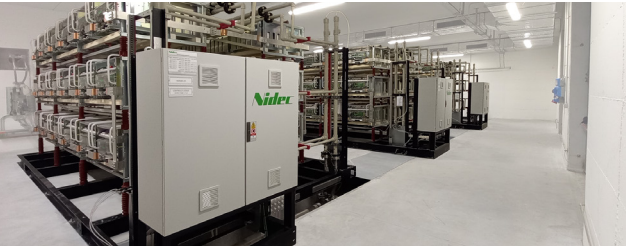
Silcovar H is a medium voltage statcom that can implement the function of “grid forming + energy storage” in delta connection configuration
