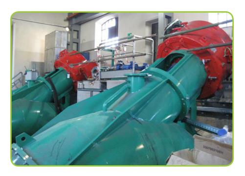
The solution: Installing Nidec Industrial Solutions permanent magnet generators
